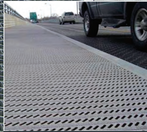
Grosse Ile Bridge, MI - Aluminum Plank Walkway
